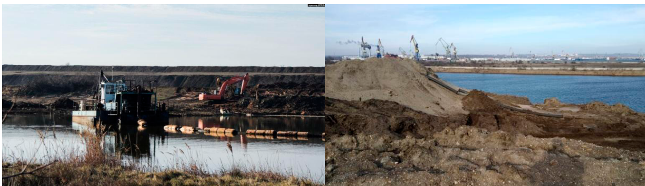
Fig. 20-21. Sand removal from the bed and banks of the bypass channel of the tailings dam with the help of a dredger in 2019. Sources: Krym.realii , Mikhail Dneprovsky (LiveJournal nordstrim).
