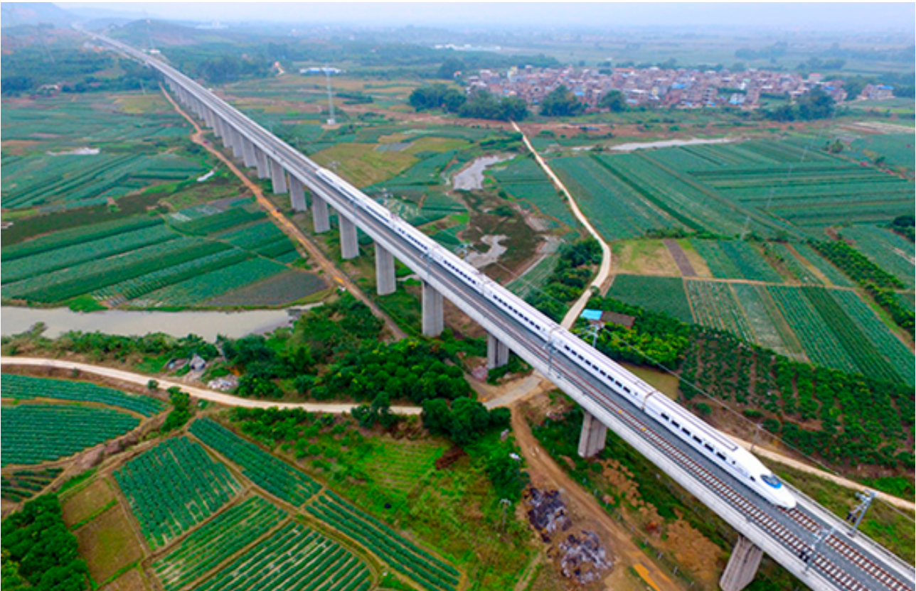
High-speed railway line through Tianyang County in China's Guangxi Zhuang Autonomous Region. Source: Wei Wanzhong / Xinhua / Globallookpress.com .
