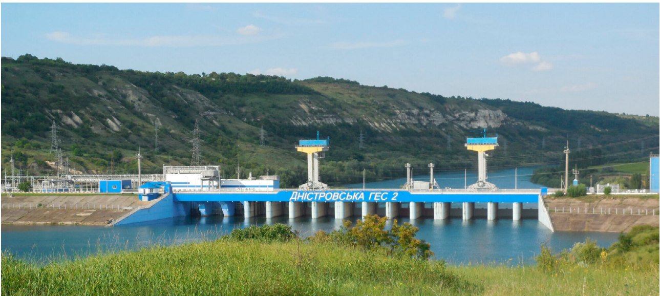
Photo 1. Dniester hydropower complex, HPP-2. Source: Ilya Trombitskiy
