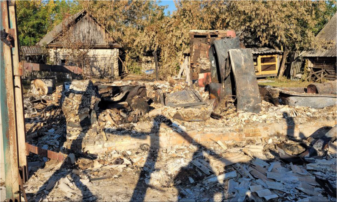
Fig. 4. The house of the inspector of the Desniansko-Starohutsky National Nature Park in the town of Stara Huta burned down as a result of shelling. Photo: Courtesy of Desniansko-Starohutsky National Nature Park Director Serhii Kubrakov.
