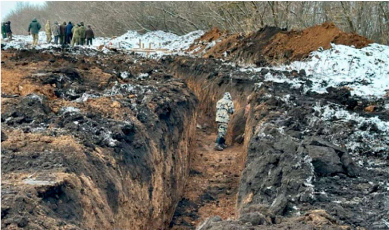
Fig. 4. Fortification construction using equipment. Photo: pravda.com.ua
