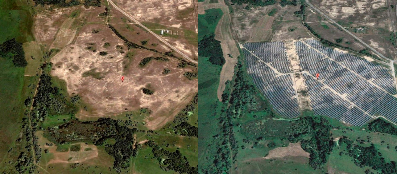
Fig. 3. The construction of a solar power plant on the sandy steppes of Lower Dnipro National Park in Kherson Oblast, as recorded in satellite images from 2018 and 2022. Source: Google Maps
