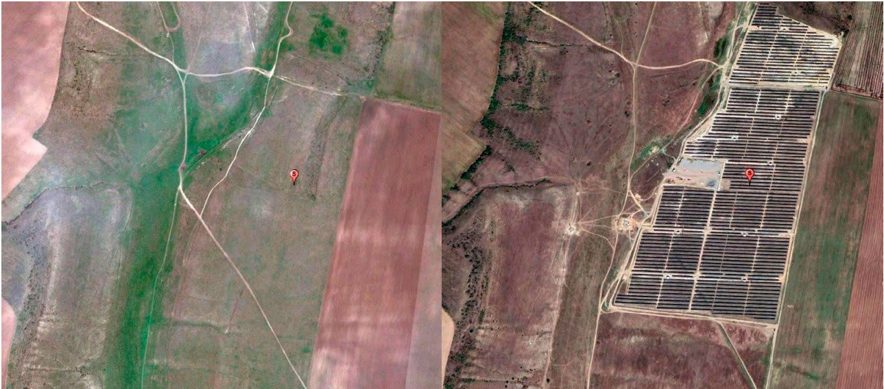
Fig. 2. The construction of a solar power plant on the slopes of a steppe ravine in the Mykolaiv region, as recorded in satellite images from 2018 and 2020. Source: Google Maps
